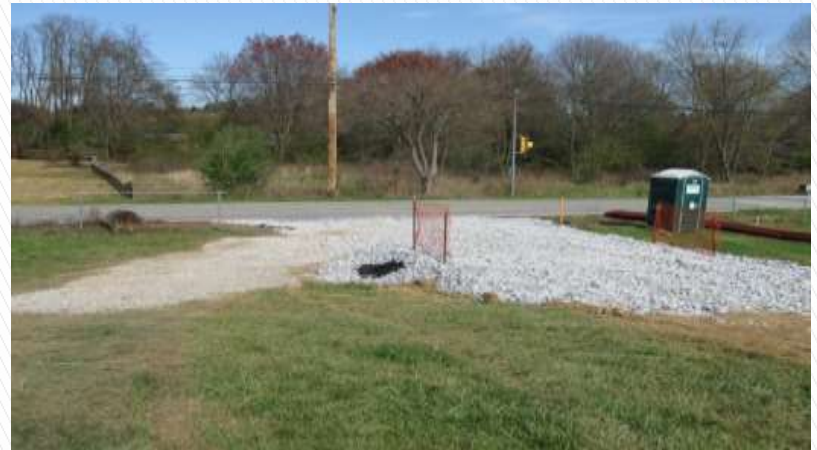
Filter Sock and Rock Construction Entrance
