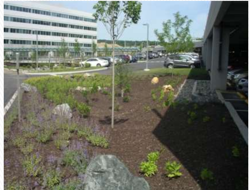
Rain Garden/ Bio Retention System
